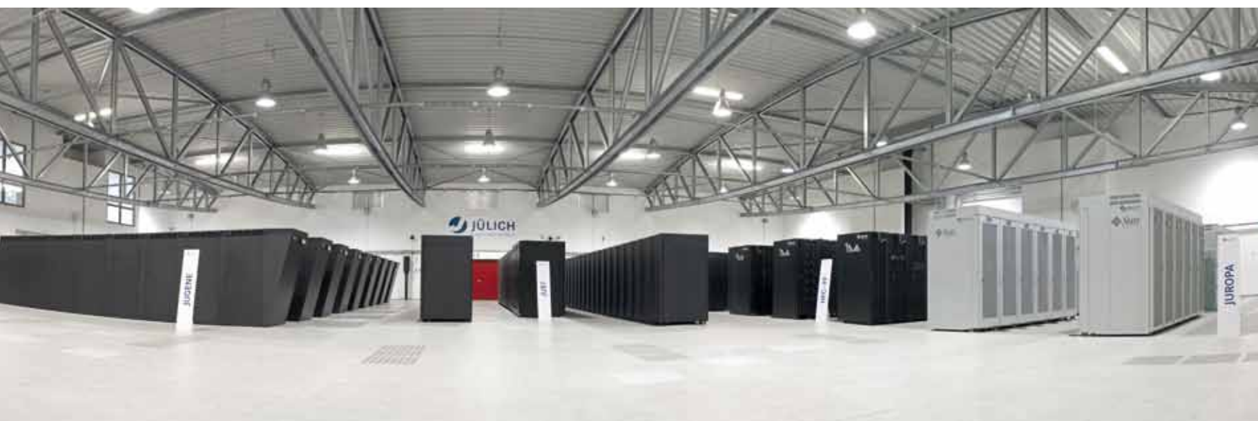
View on the supercomputers JUGENE, JUST (storage cluster), HPC-FF and JUROPA in Jülich (Photo: Research Centre Jülich)
