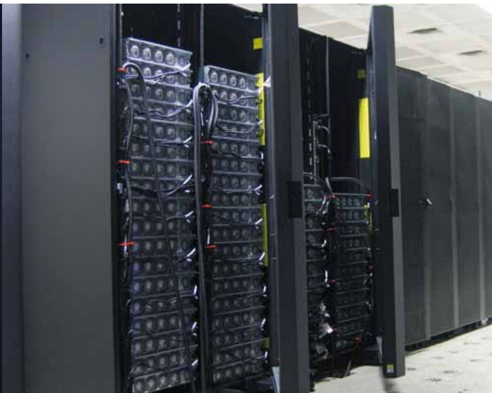
Figure 2: Back side with rear door heat exchanger
